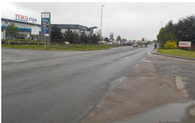
Figure 10 - View looking north on Cromwell Road
