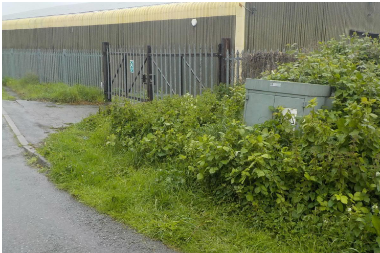
Figure 6 - Existing sub-station on New Bridge Lane
